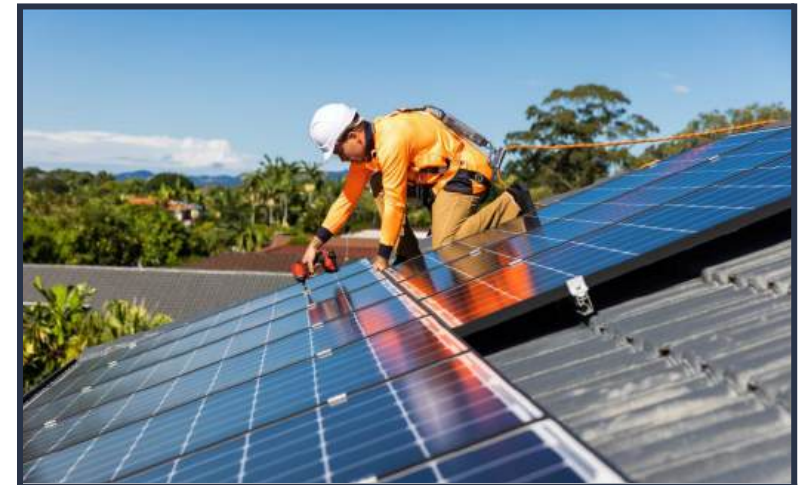
Figure CRI.2: Solar panels being fitted to an existing roof. Credit - Canva
